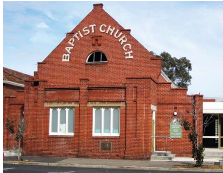
ABOVE: St Kilda Baptist Church on Pakington Street.
